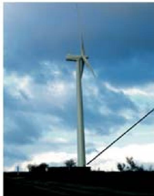
Figure 6 Position of a wind turbine at the crossroads of fault zones
